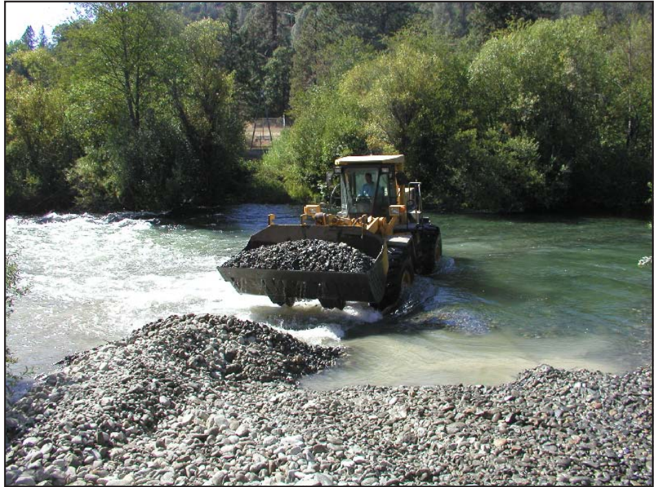
Gravel was placed directly in the Trinity River by local contractor Clint Robison
