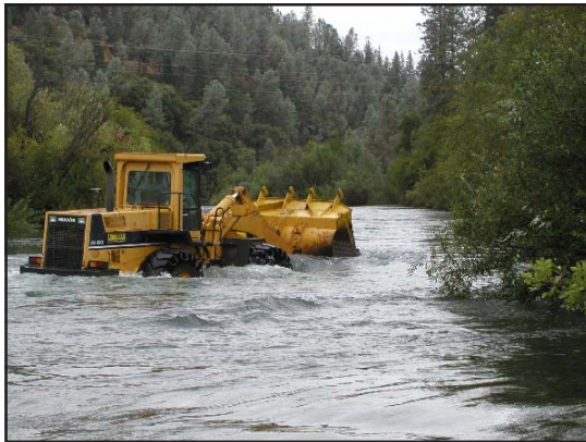
Gravel was spread to an approximate in-river depth of one or two feet
