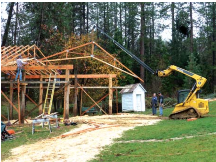
Pavillion during construction.
