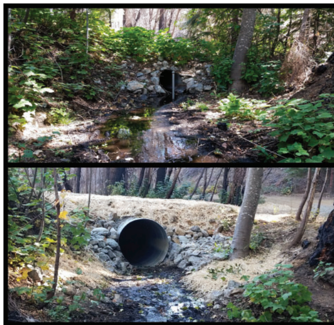
Culvert replacement project at Hocker Meadow Creek
