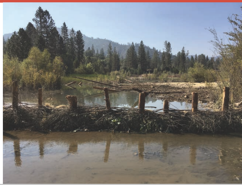
A beaver dam analog constructed at the Bucktail Restoration Site in Lewiston
