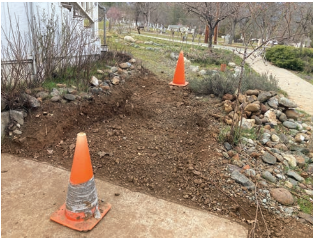
Before sidewalk construction
