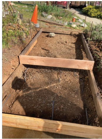
During sidewalk construction
