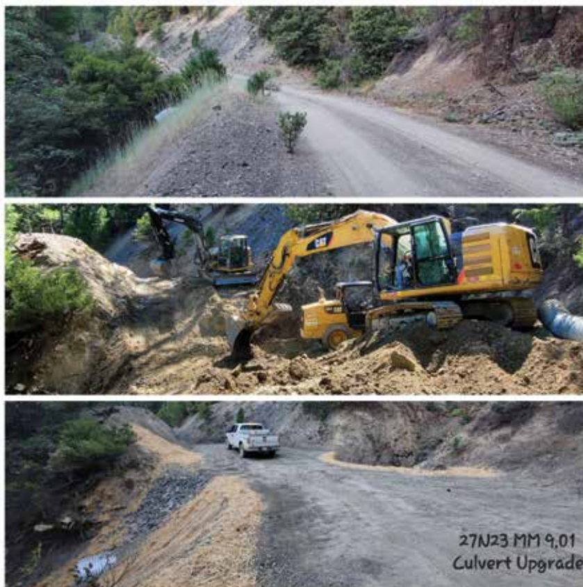
Culvert upgrades on the 27N23 road that leads to a Yolla Bolly-Middle Eel Wilderness trailhead.
