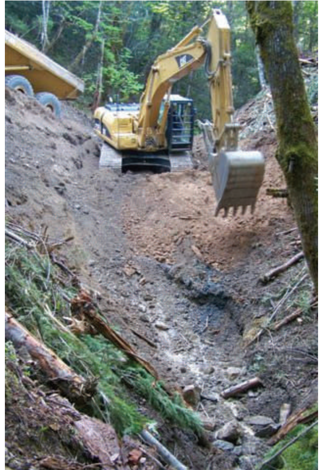
Road decommissioning of 4N15 road at Mile Marker 1.07
