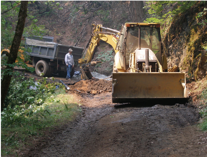
Union Hill Road Upgrade
