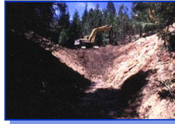
Heavy Equipment Work-Landing Removal
