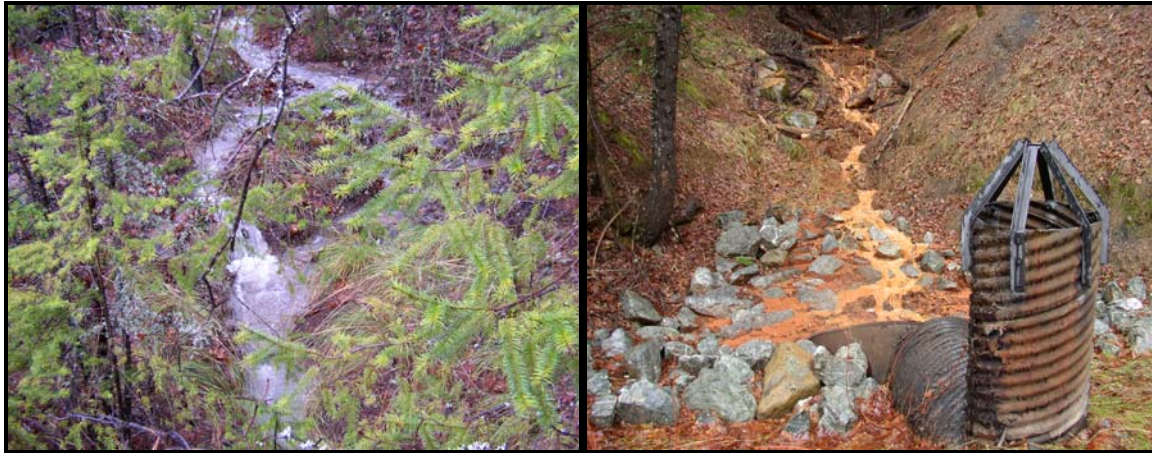
Photo 5-1 Inlet of culvert at mile marker 62.13 and 61.81
