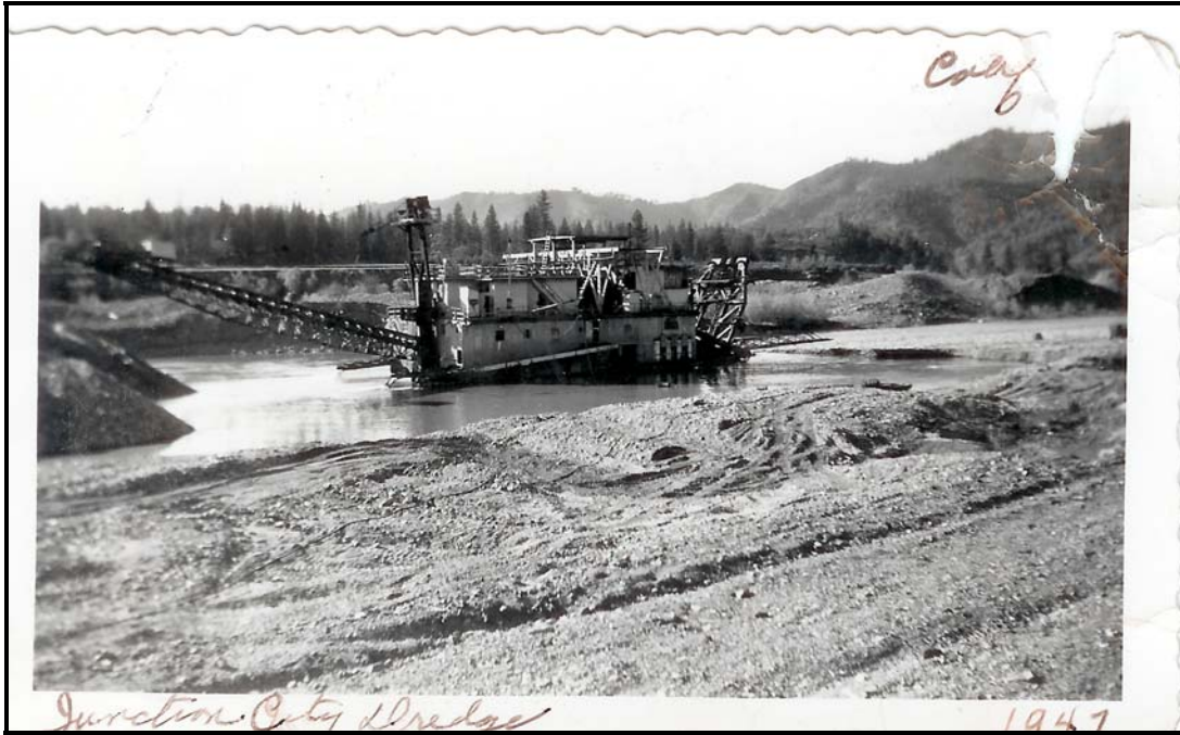
Photo 3-1 Typical bucket line dredge used along the upper Trinity River leaving piles of dredge tailings. This photo was taken in 1947 in Junction City.
